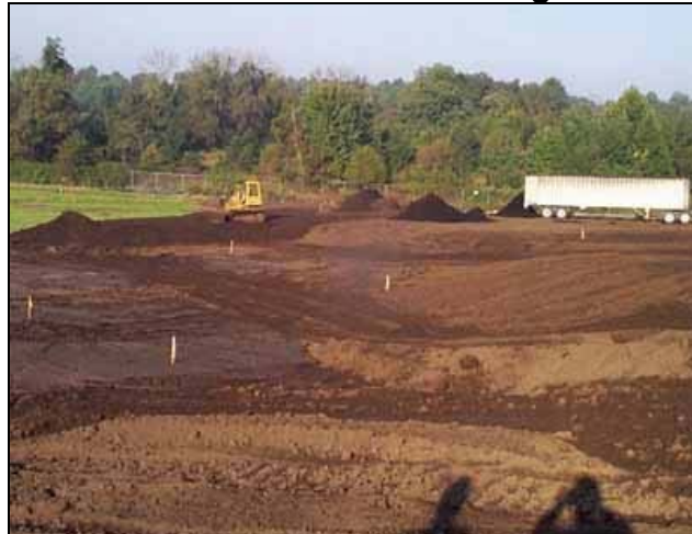
Figure 6-1. Wood Treating Site: On-site Thermal Desorption of Contaminated Soils. Final Grading and LeafGro® Placement
